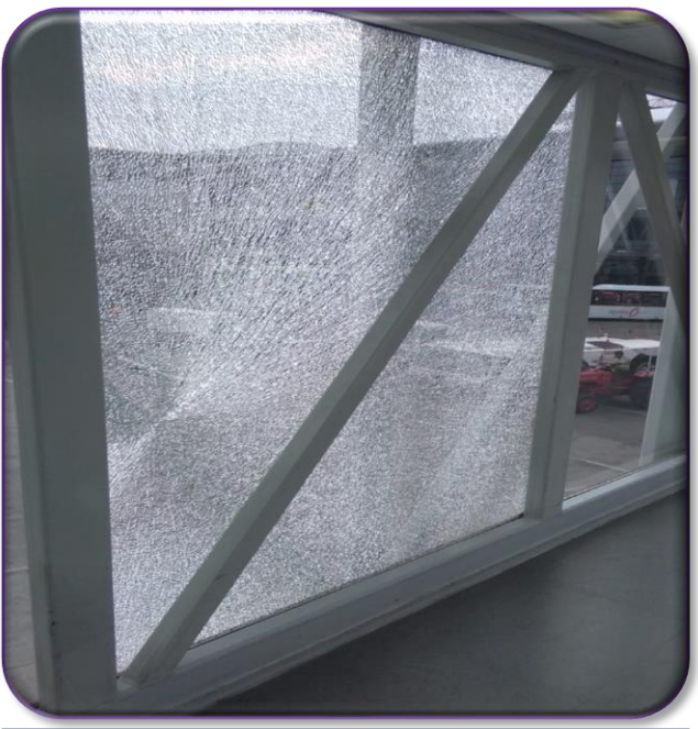
Tunnel glass Damage
